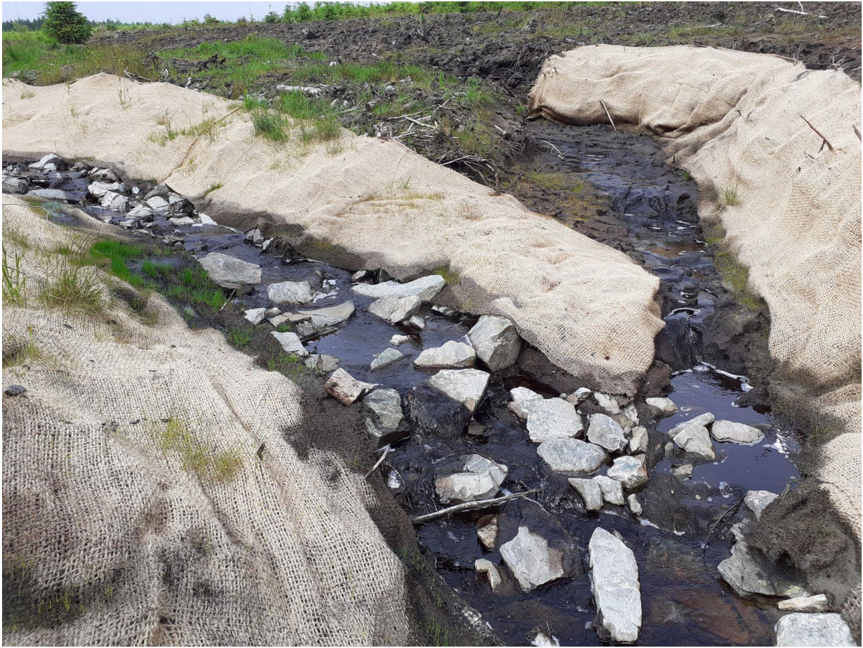
Photo 4- confluence of stream from Wall 3 & Sruhingarve stream, 8/7/22
